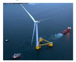
25 MW (3 x 8.4 MW)20km off-shore100m depth
