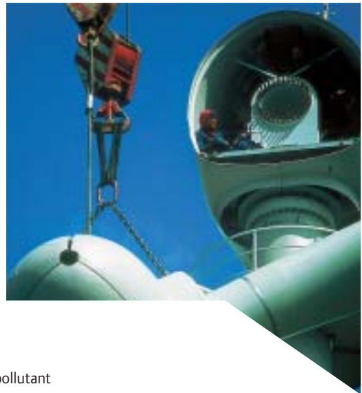
Fonte da Mesa – Installing wind turbine.
