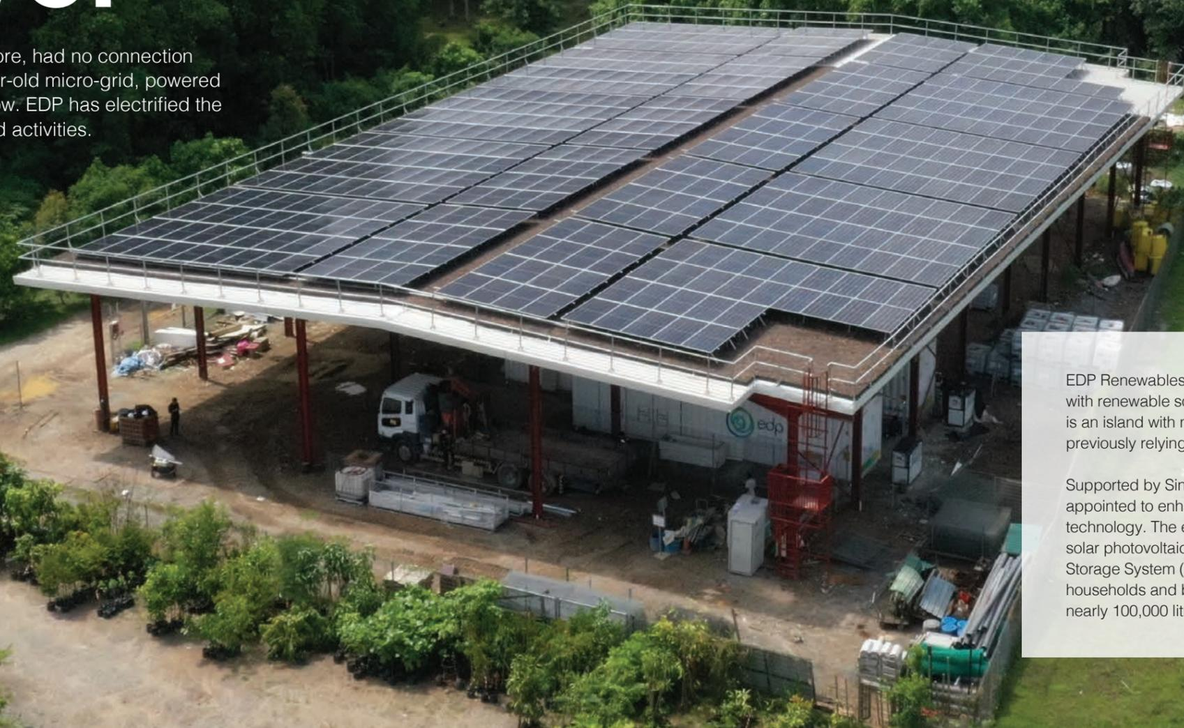
EDP Renewables in APAC has recently greened Pulau Ubin's Micro-grid with renewable sources. Situated to the north of Singapore, Pulau Ubin is an island with no connection to the mainland's power grid and was previously relying heavily on diesel.
