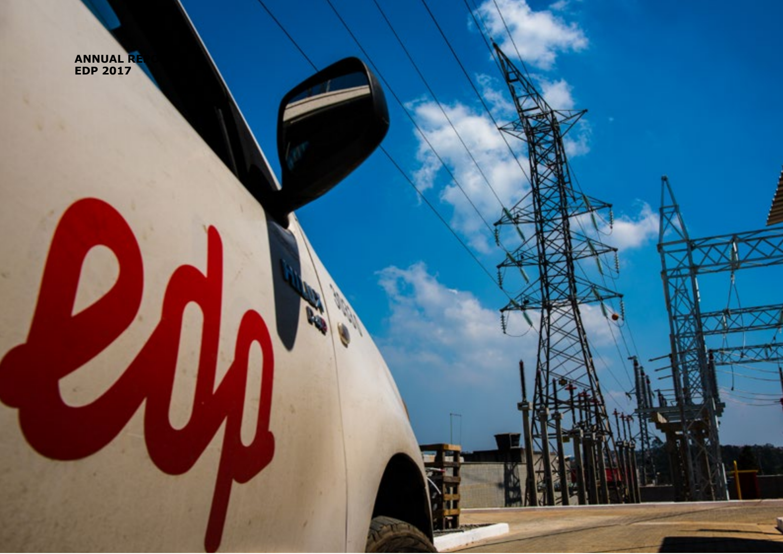
EDP São Paulo Substation in Biritiba Mirim
