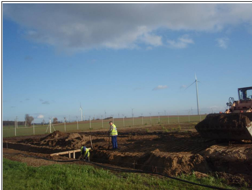
Photo 8: The electrical substation in Sypniewo – installation of the underground cables.
