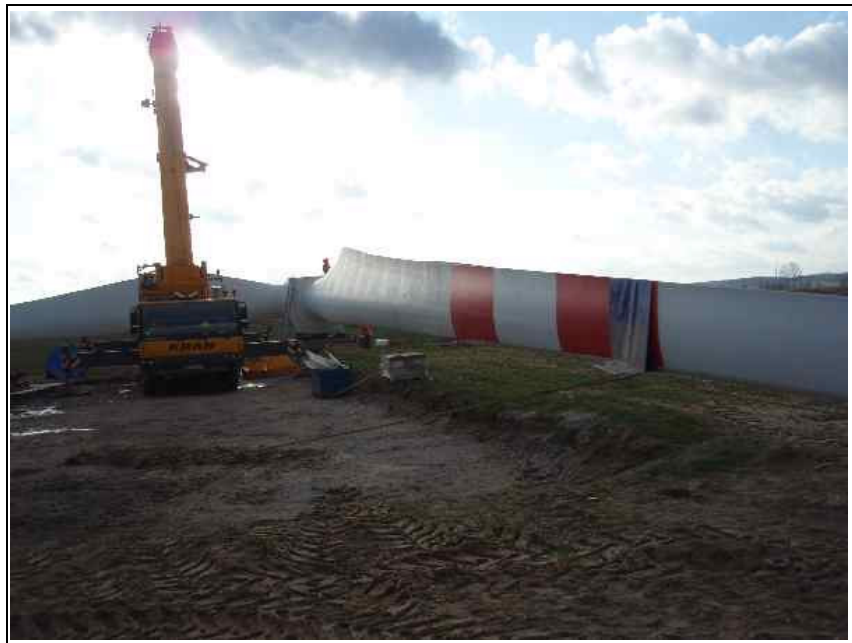
Photo 6: The blades are assembled before mounting on the top of the tower.
