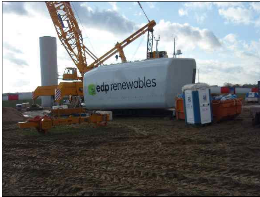
Photo 5: The wind turbine elements are large (a gondola)
