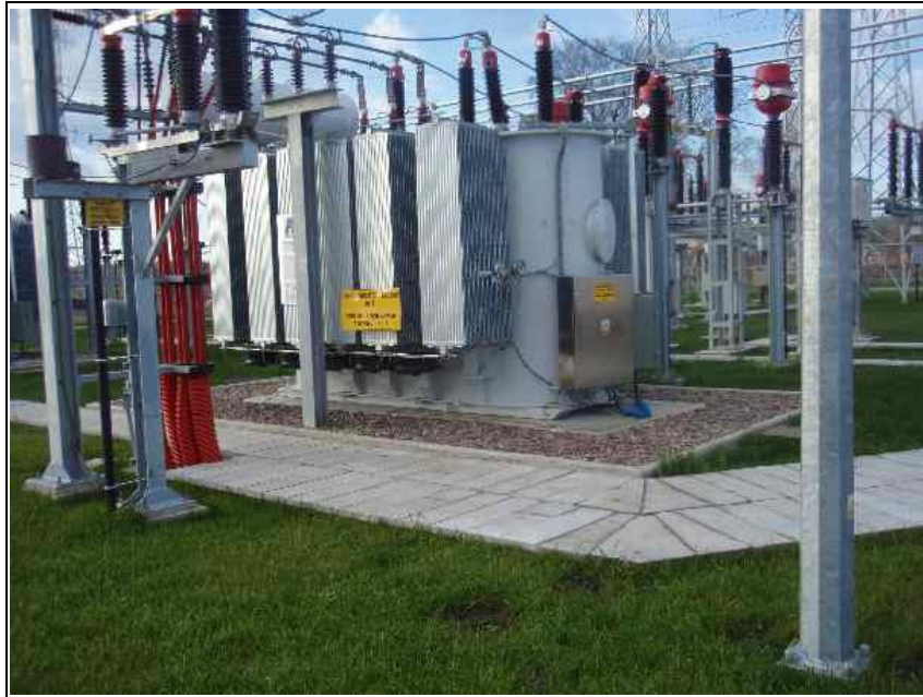
Photo 7: The electrical substation in Sypniewo – a transformer on a secondary containment.
