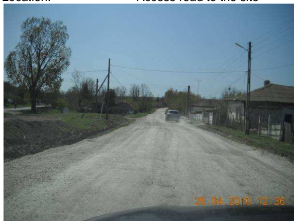
Access road condition: compacted gravel road
