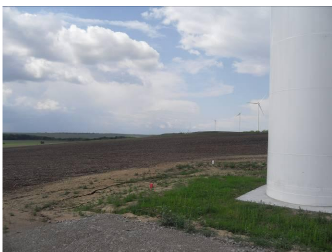
Figure 8 – View from base of turbine 7
