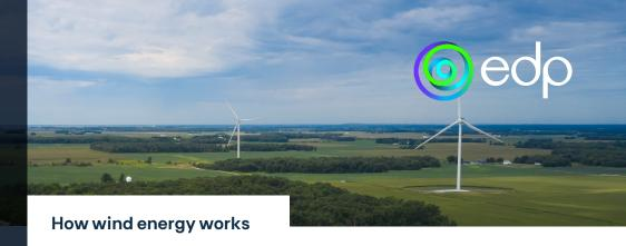
EDPR NA uses wind turbines to harness the natural resource of wind to generate mechanical energy. This energy is transformed into electricity via a generator and is sent to the electrical grid after being converted to the proper voltage.
