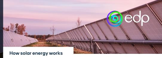
EDPR NA uses photovoltaic (PV) solar cells. Photovoltaic solar cells have no moving parts and convert sunlight directly into electricity via the photoelectric effect. This direct–current electricity is then collected, transformed into alternating current, and finally put on the electrical grid through a substation after being converted to the proper voltage.
