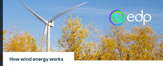
EDPR NA uses wind turbines to harness the natural resource of wind to generate mechanical energy. This energy is transformed into electricity via a generator and is sent to the electrical grid after being converted to the proper voltage.
